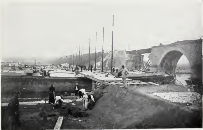
CONSTRUCTING A BRIDGE OF BARGES ON THE MARNE
